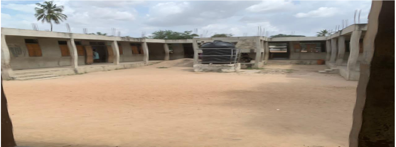
CONSTRUCTION 12-UNIT CLASSROOM BLOCK WITH OFFICE AND STORE AT KOTOKU – PHASE 1
