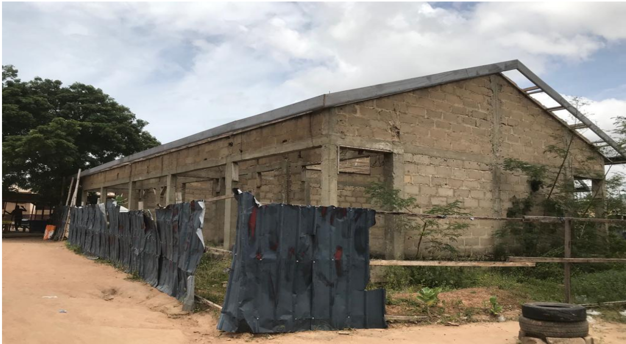
CURRENT STATE OF THE PRE -SCHOOL PROJECT AT NSAKINA
