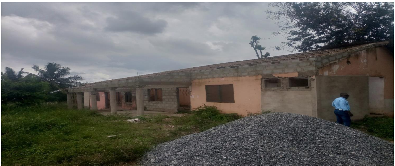
MAYERA HEALTH FACILITY- PRESENT STATE
